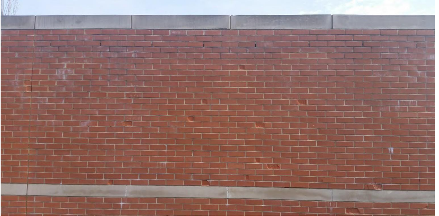
Intermediate School Wall next to Loading Dock
