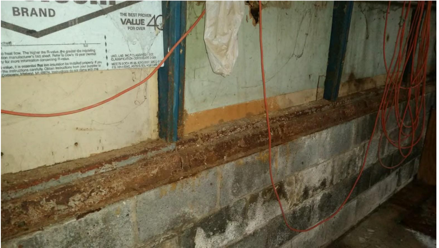
Cinder/Batting Shed – Insulation and decay.
